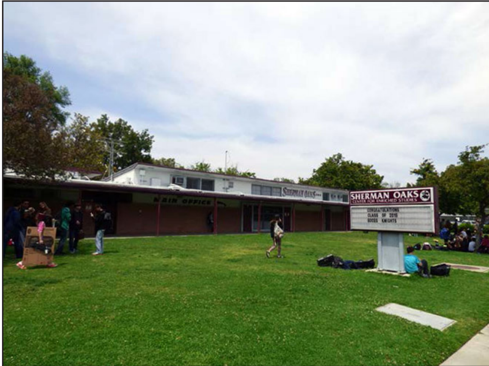
Photo 1. View looking Northeast toward front school entrance and main office.
