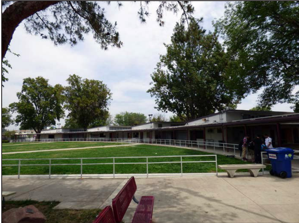
Photo 3. View looking East toward Central Courtyard and Classroom Buildings in Southeast Portion of Campus.
