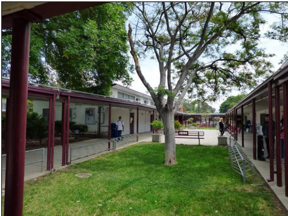
Photo 2. View looking North toward courtyard between the Library and Administration Buildings.
